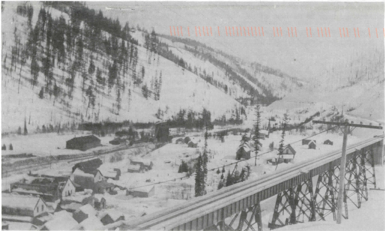
Saltese MT, looking east, just after the steel bridge had replaced the wooden trestle. March 14, 1911. The NP line over Lookout Pass is to the left, at grade level. Notice there does not appear to be any sort of road in evidence at this time. Photo in MilWest Archives.
